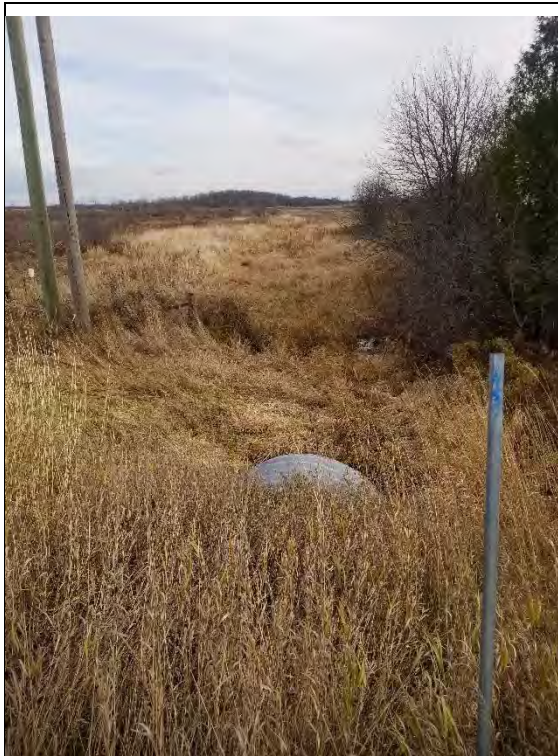
Photo 1: Gordon Drain downstream of culvert at Highway 12. Facing east.
