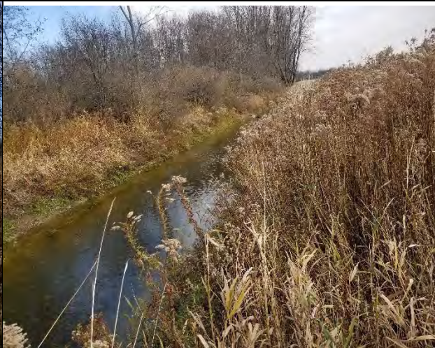
Photo 4: Gordon Drain downstream of Lot 13. Clean out completed within last 5 years +/- . Bed and banks free of vegetation to top of water. Ditch is well defined with approximately 0.75 m standing water.
