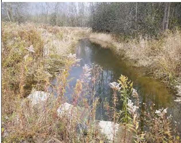
Photo 5: Crossing through drain at west side of Lot 15. Four- 1 m rise x 650 mm span structural plate corrugate steel arch culverts.
